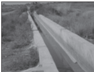
Al Dahra concrete water course in village Sayed Ali Nawaz Shah
