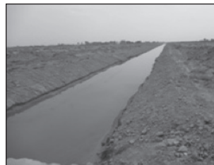
New water channel sanctioned from Irrigation Department of Sindh for Al Dahra Grass fields
