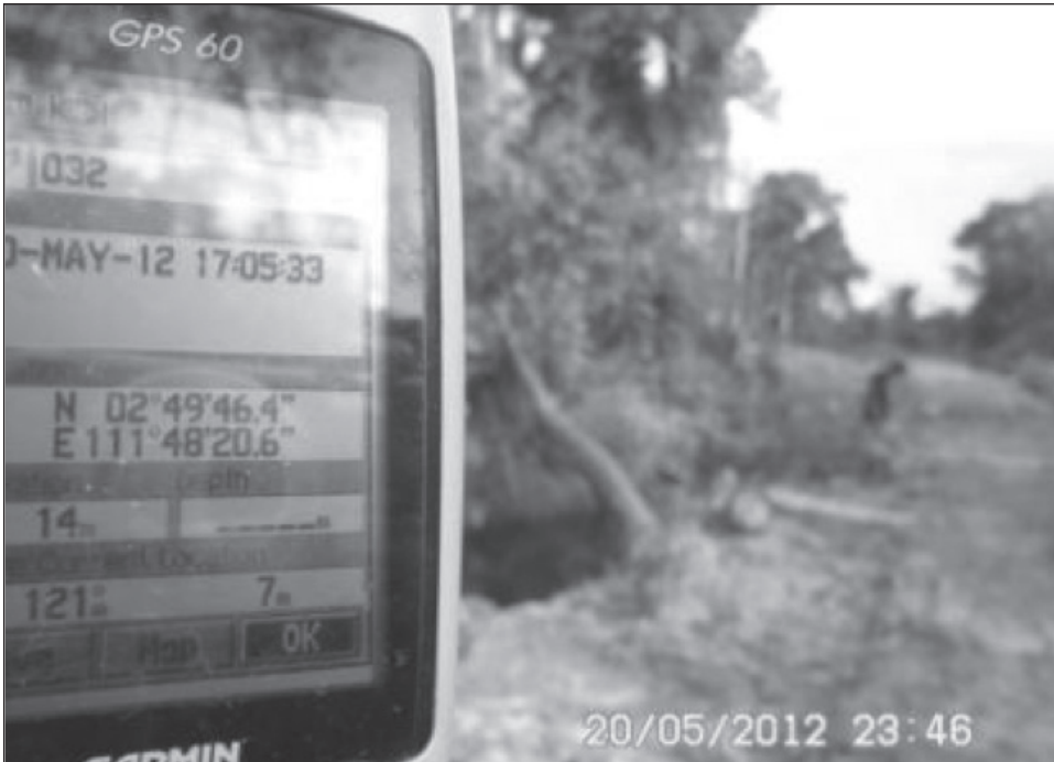
N 02 49' 46.4" E111 48' 20.6"(Point GPS). Ilas River is badly damaged due to road construction by Sarananas Sdn. Bhd., which blocked the river.
