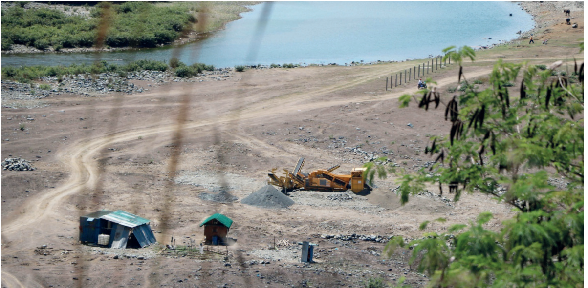
Image 6. Ongoing construction of the Balog-balog dam
